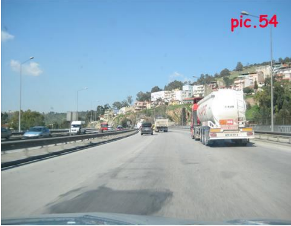
Pic.54: Bridge crossing on D-550 road - Carriage capacity 600t
