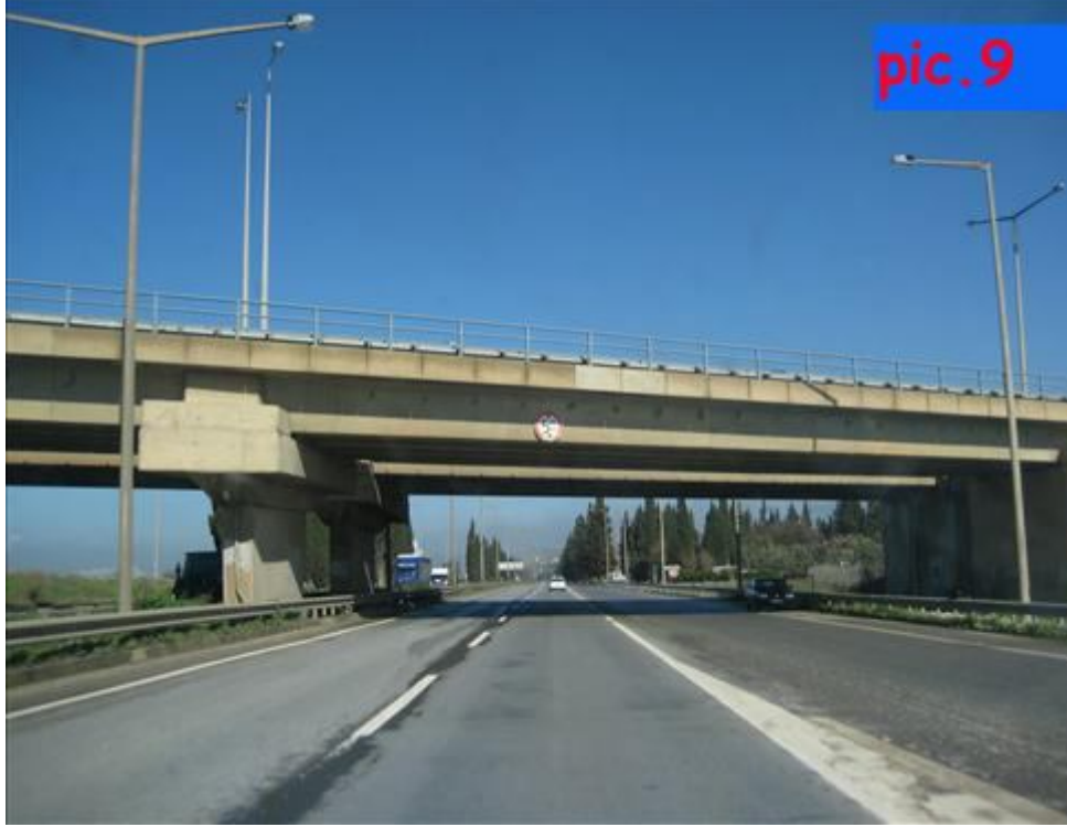
Pic.9 : Highway bridge. Height (m) is aprox. 5,2 meter. -D-550
