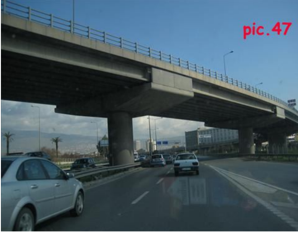
Pic.47: Subway under highway bridge on road 35-51
