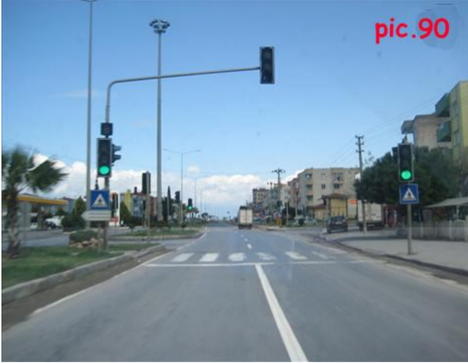
Pic.90: Traffic signal on D-550
