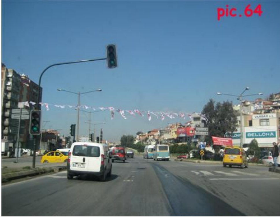
Pic.64: Traffic signals on D-550
