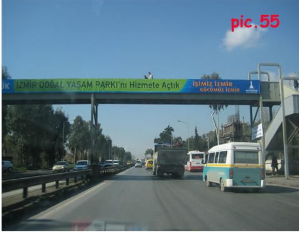
Pic.55: Footbridge on D-550 road.
