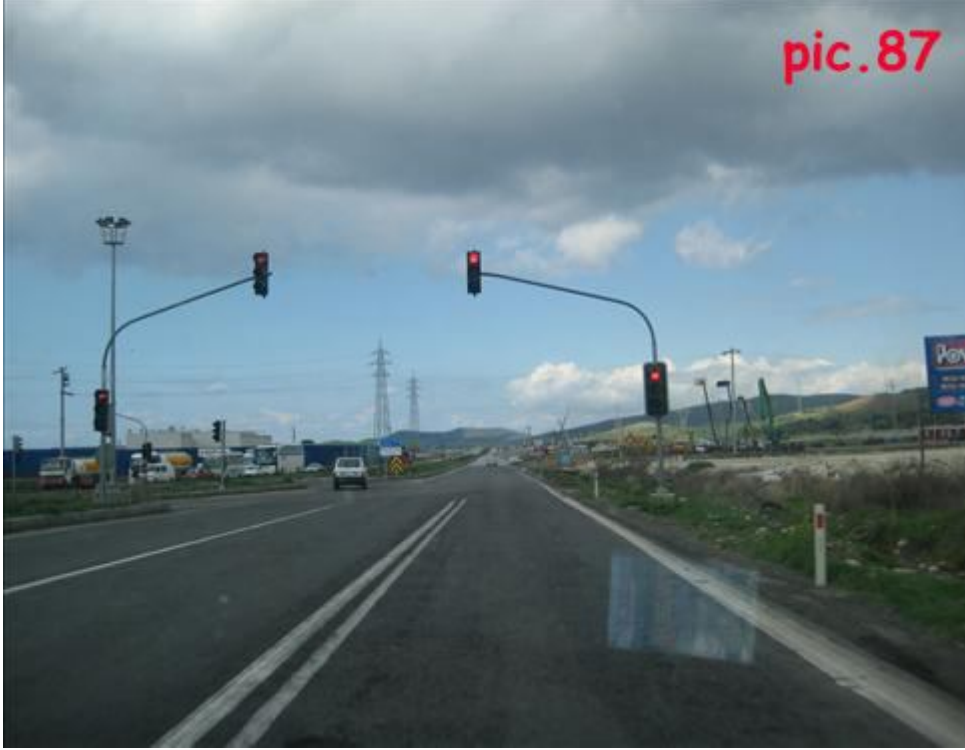
Pic.87: Traffic signal on D-550
