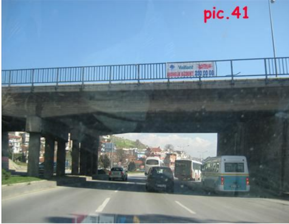
Pic.41 : Subway passing under highway on road 35-51
