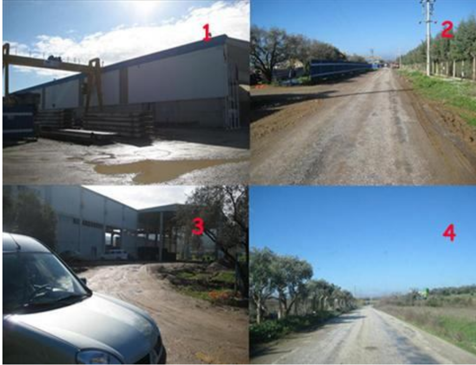
Pic.1: Arkas loading area. Pic.2: Narrow road in front of Arkas factory. Pic.3: Arkas factory Pic.4 : Narrow road between arkas factory to bridge.
