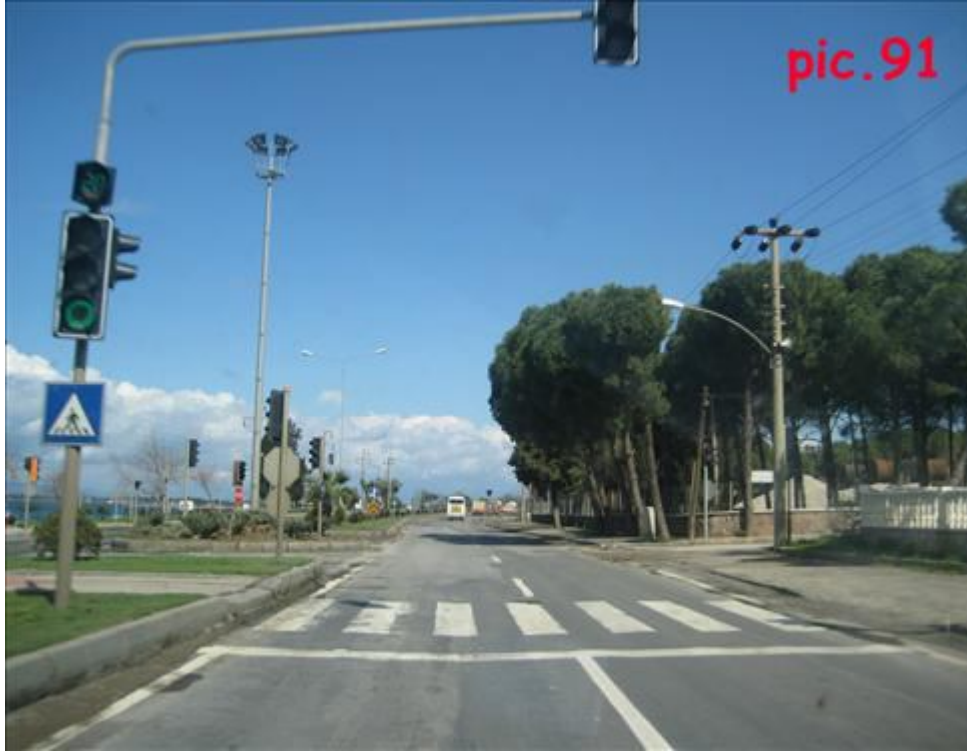
Pic.91: Traffic signal on D-550
