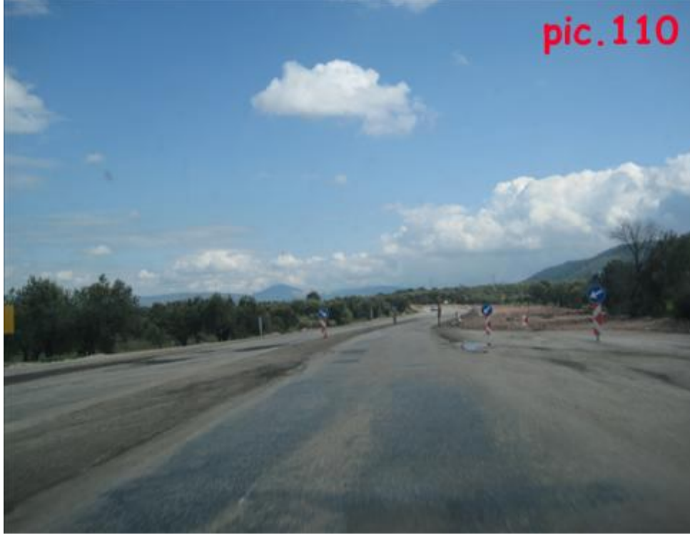
Pic.110: Road construction -Width of road: 4,5 m
