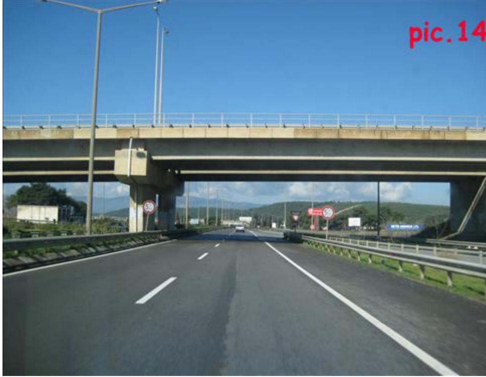
Pic. 14: Subway passing under highway bridge.
