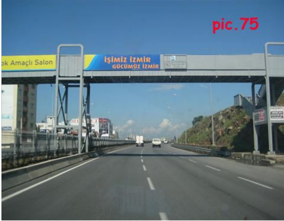
Pic.75: Footbridge on D-550
