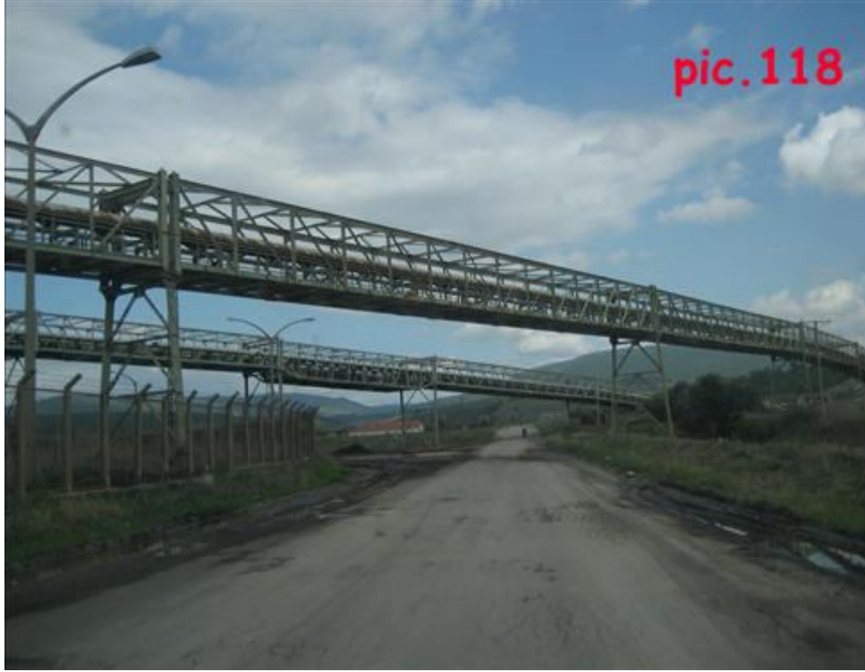
Pic.118: Two conveyor line.
