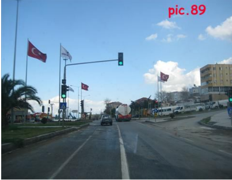
Pic.89: Traffic signal on D-550
