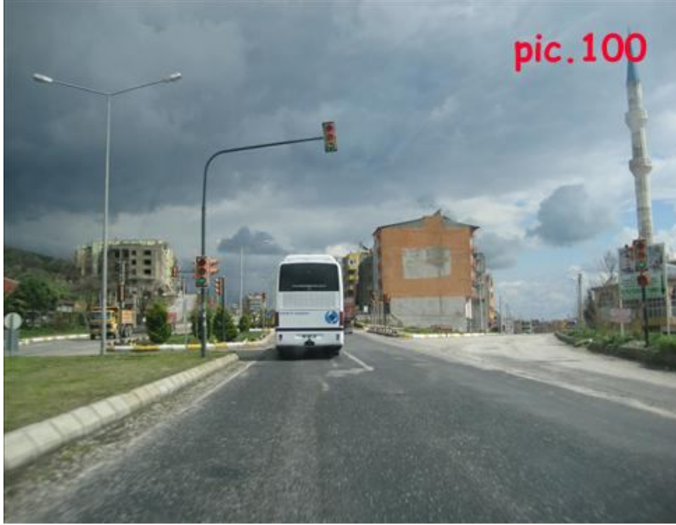
Pic.100: Traffic signal on D-240
