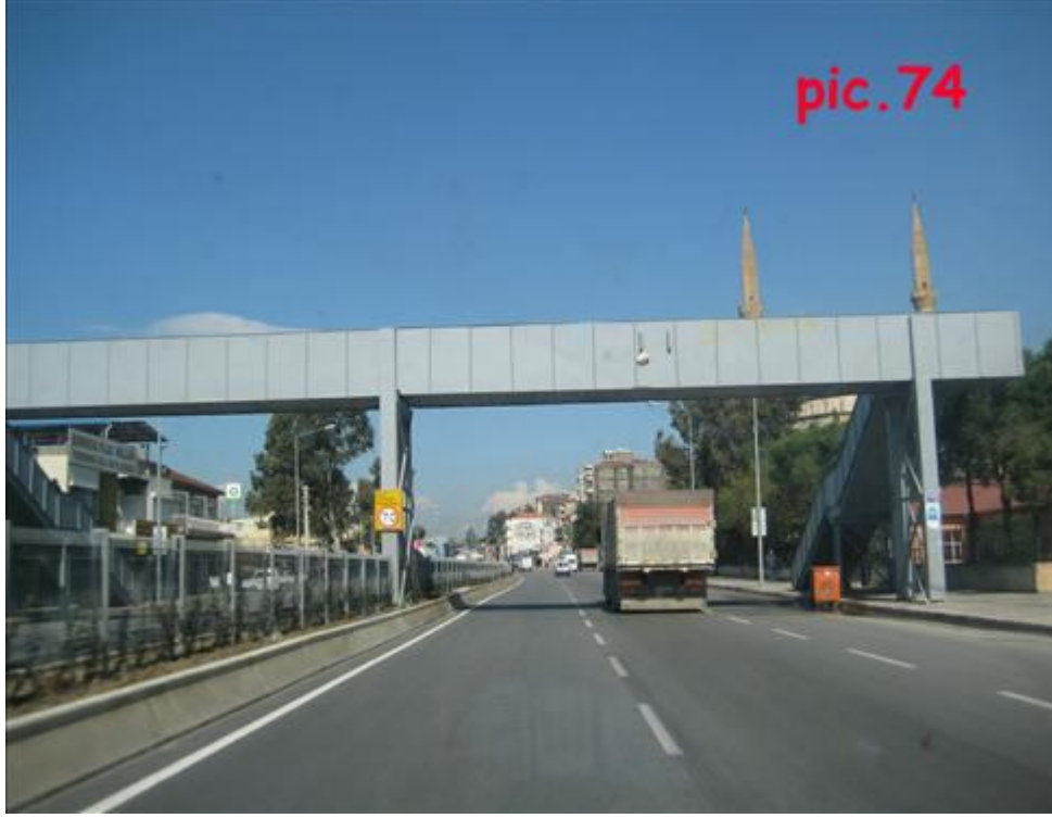
Pic.74: Footbridge on D-550
