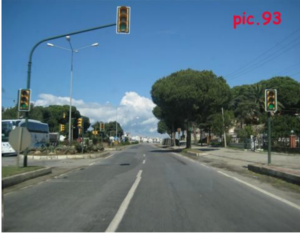
Pic.93: Traffic signal on D-550
