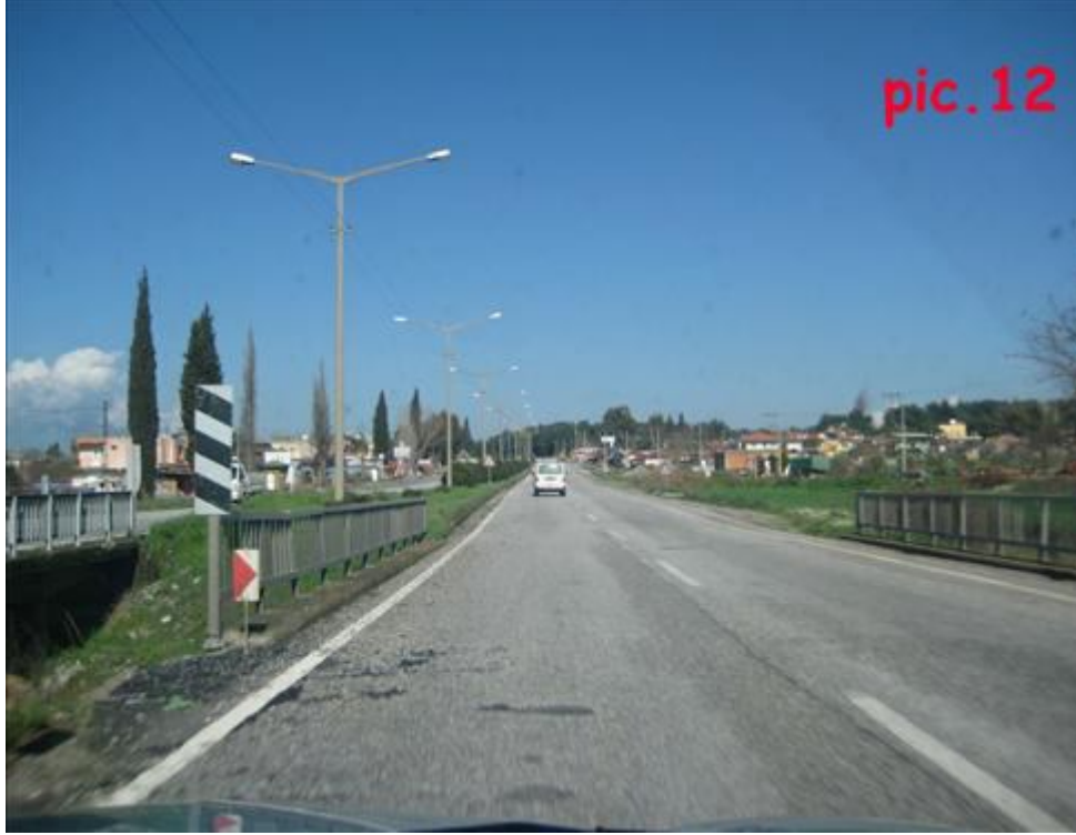
Pic.12: Bridge crossing. Width 10 meters -Length (m) : 20 meters -Capacity of Bridge: 520t
