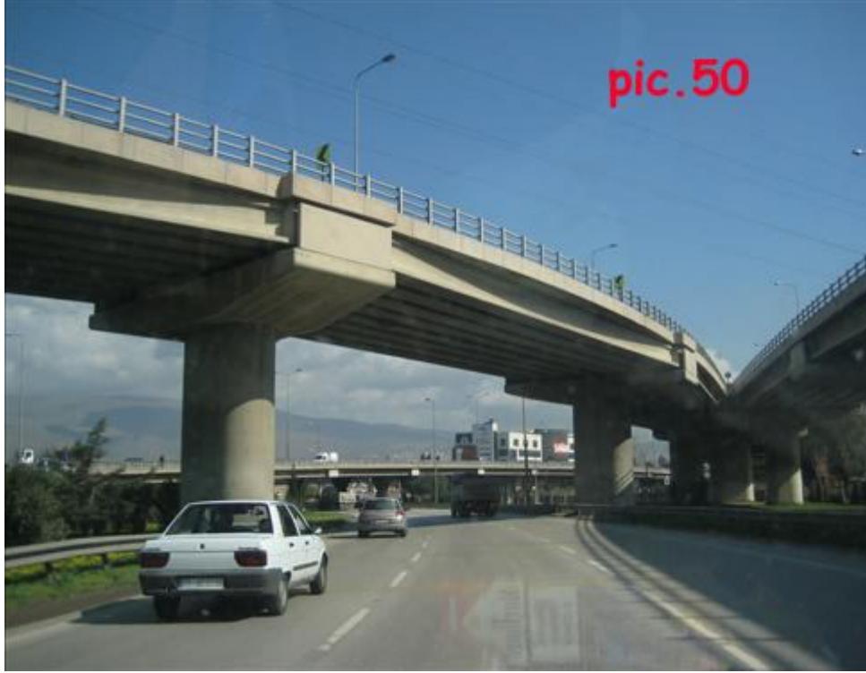
Pic.50: Subway passing under highway bridge on road D-550
