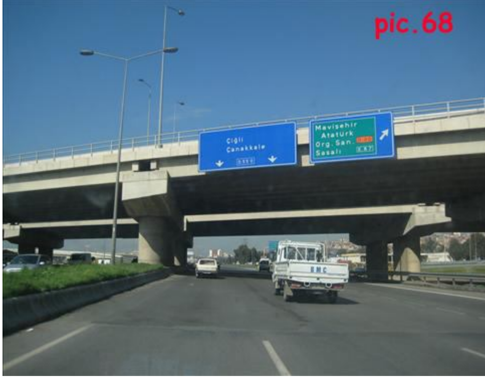
Pic.68: Highway bridge on D-550
