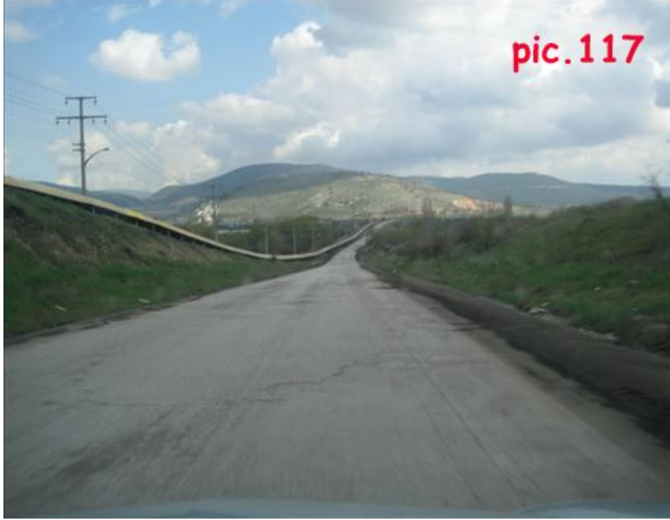
Pic.117: Energy plant next to left to Accessing site area narrow road starts
