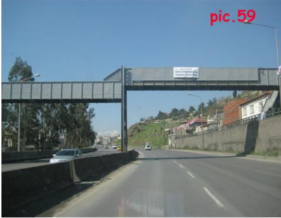
Pic.59 : Footbridge on D-550 road
