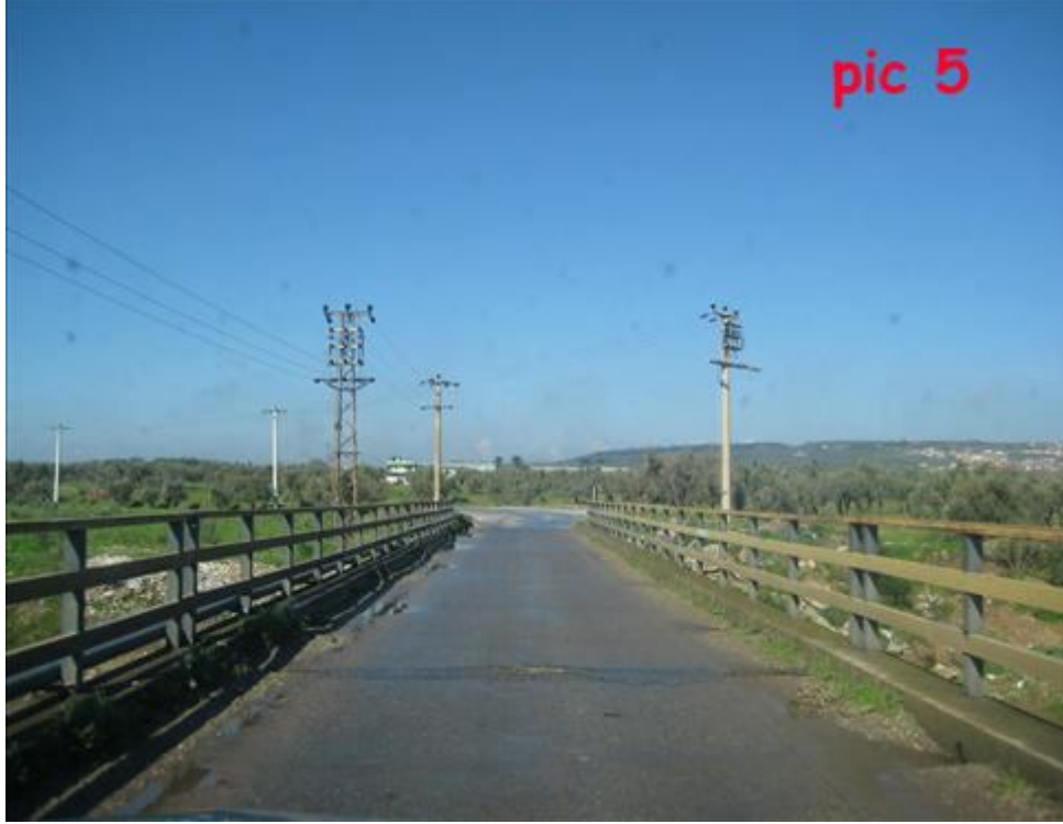
Pic.5: Bridge near the Arkas factory -Capacity of Bridge: 45 t/axle
