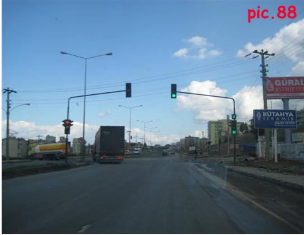
Pic.88: Traffic signal on D-550
