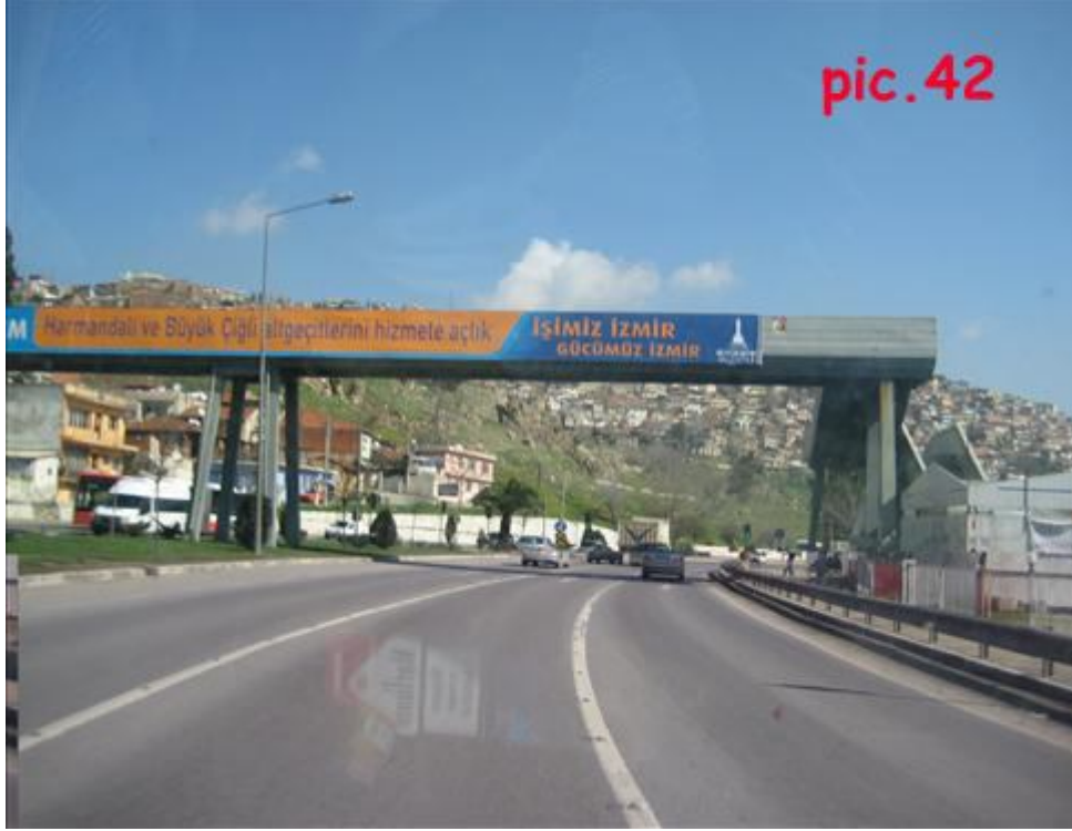
Pic.42: Footbridge on road 35-51
