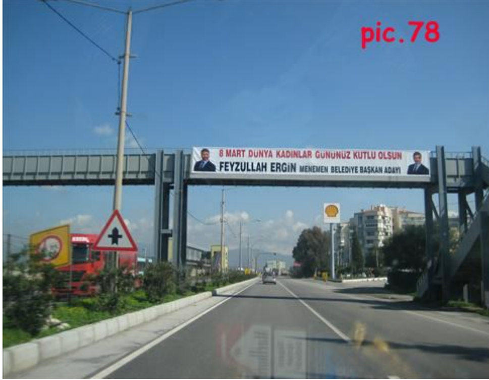
Pic.78: Footbridge on D-550
