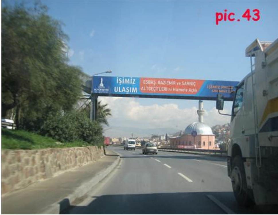
Pic.43: Footbridge on road 35-51
