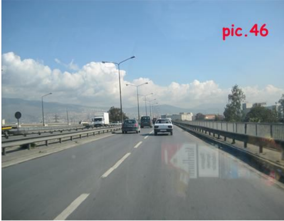
Pic.46: Viaduct crossing. On road 35-51. -Lifting capacity of viaduct 600 t
