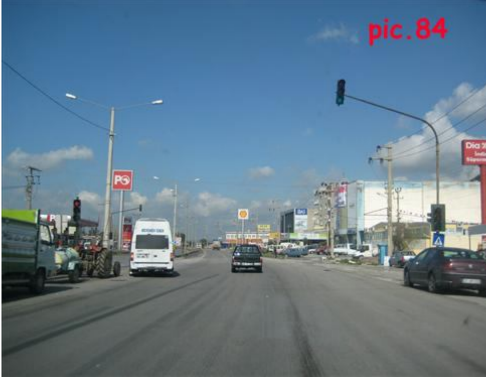
Pic.84: Traffic signal on D-550
