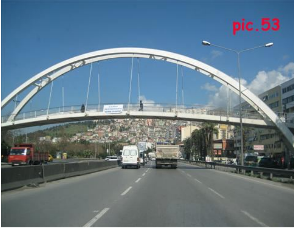
Pic.53: Footbridge on road D-550.
