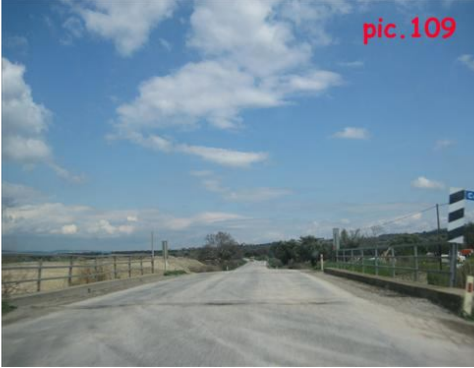
Pic.109: Bridge crossing
