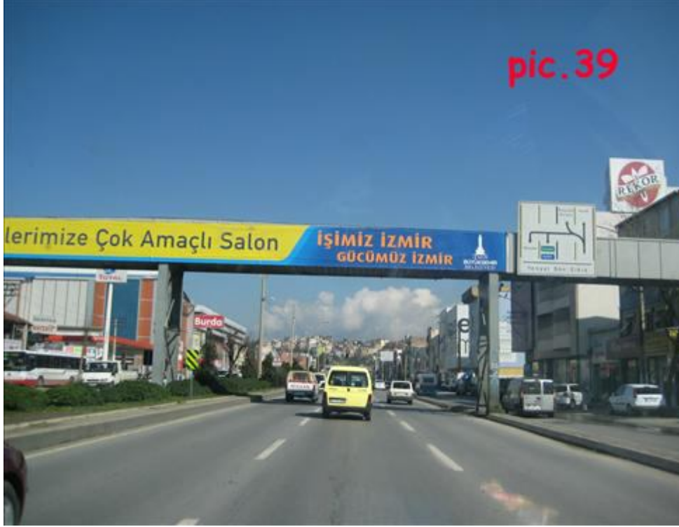
Pic.39: Footbridge on road 35-51
