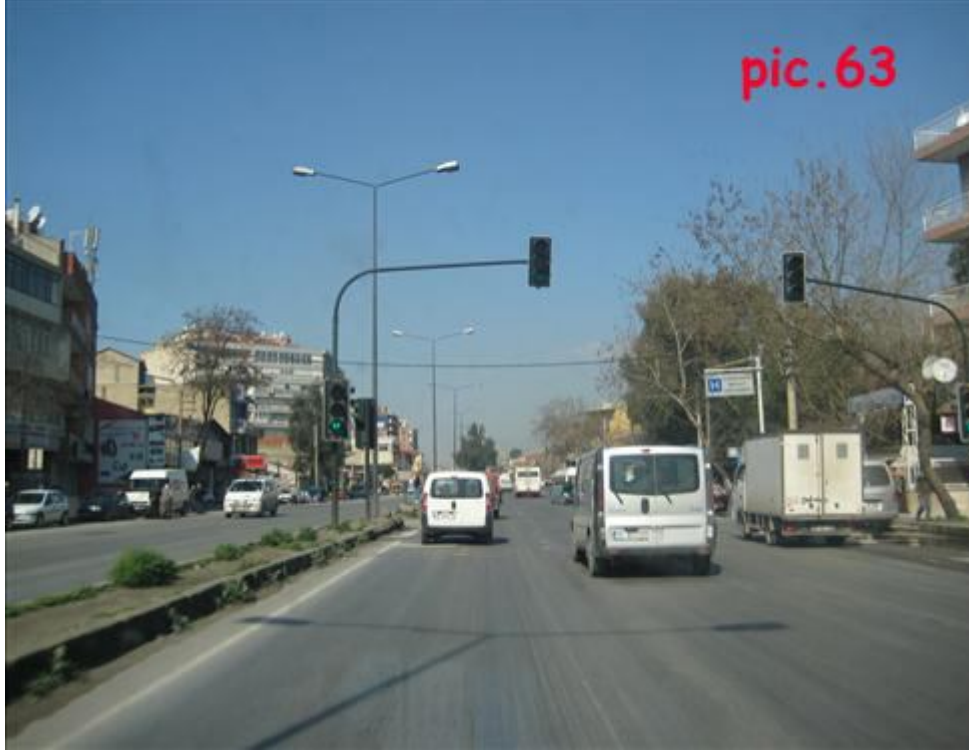
Pic.63: Traffic signals on D-550
