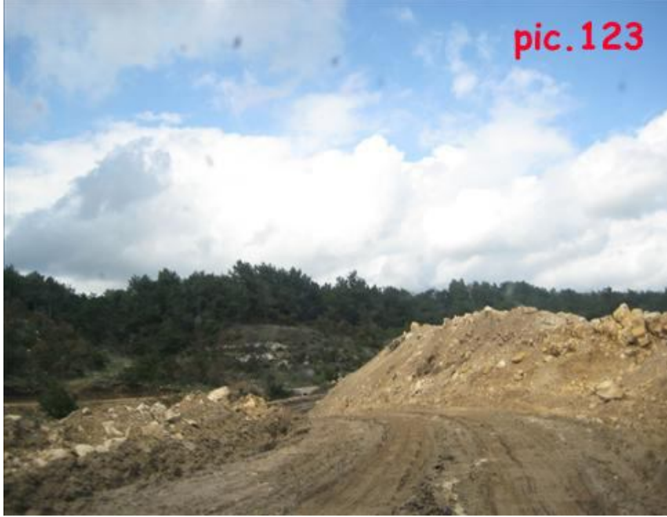
Pic.123: Narrow ,dirt damaged road. -Begining of forest
