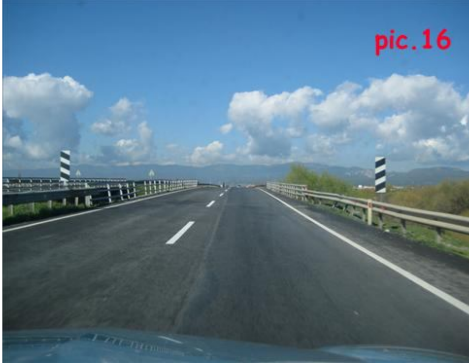
Pic.16: Bridge crossing Bridge dimension
