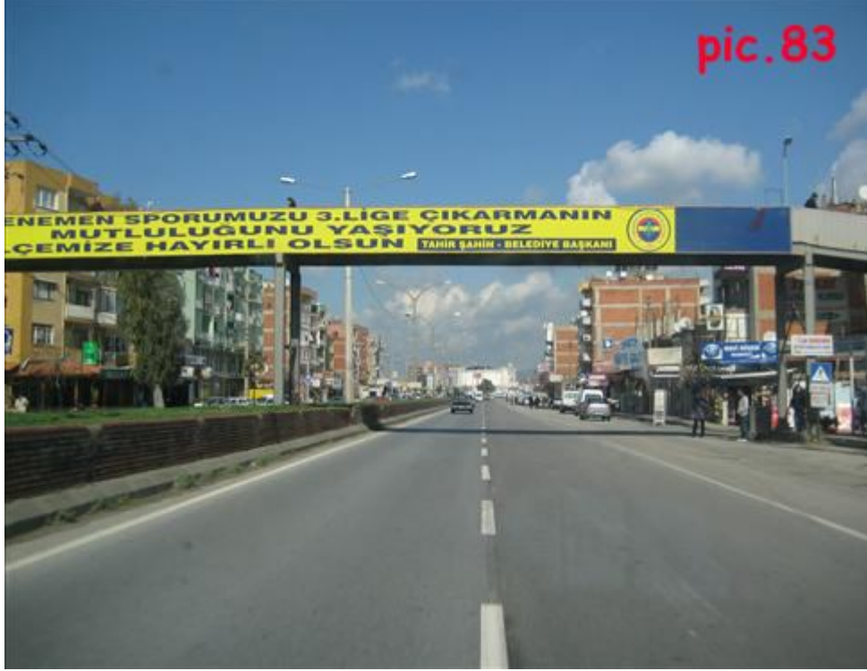
Pic.83: Footbridge on D-550
