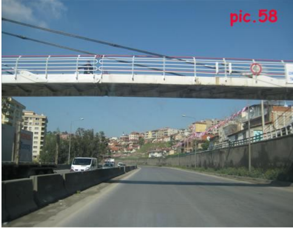
Pic.58 : Footbridge on D-550 road
